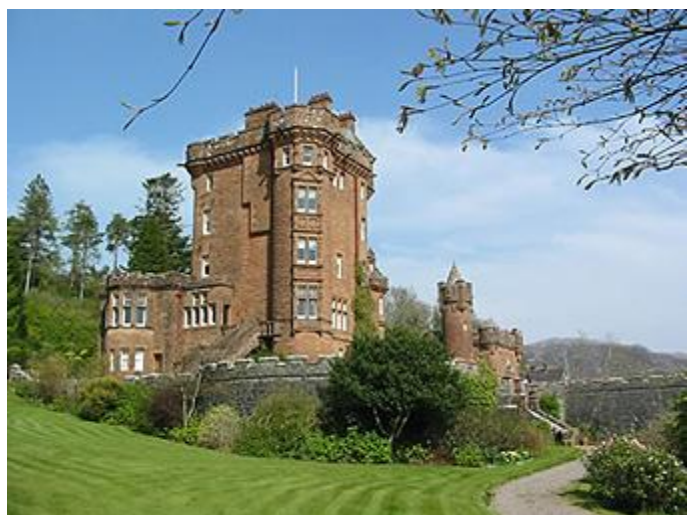
Glenborrodale Castle, Ardnamurchan, Argyll
